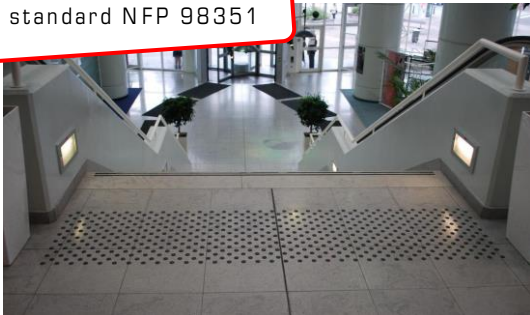
Installed on marble
